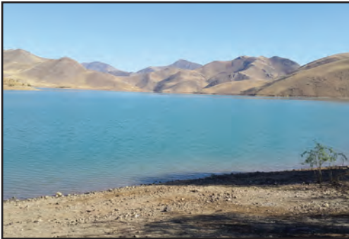
Plate 3. A view of Gavoshan dam. © Loghman Maleki
