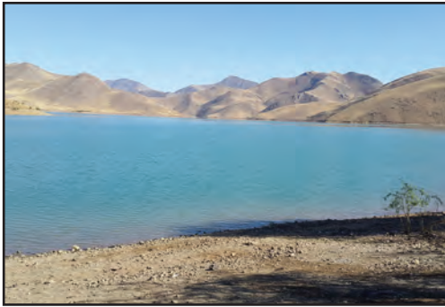
Plate 3. A view of Gavoshan dam. © Loghman Maleki
